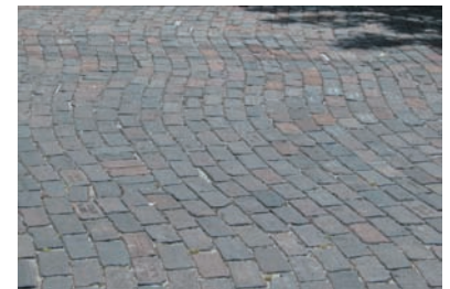
FIGURE 5.20 The bricks were originally straight. Do you see the evidence for cars pushing backward on the road as they accelerate forward? Or pushing forward on the road as they brake?
