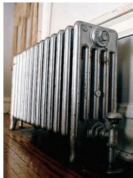
FIGURE 17.6 Internal energy is released by steam when it condenses inside the “radiator.”
